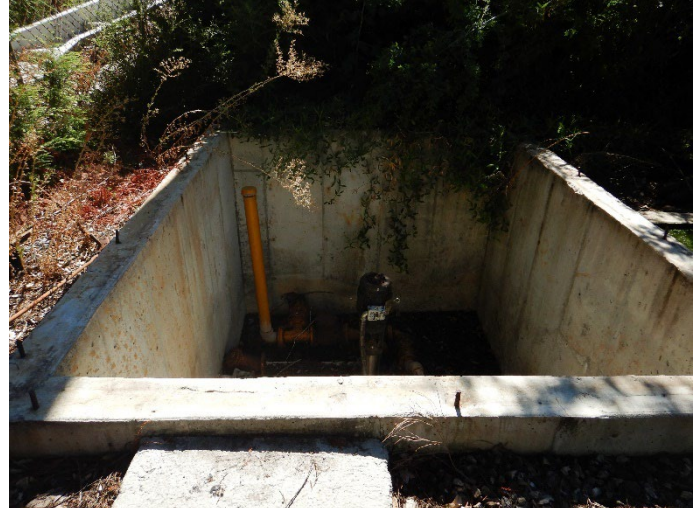
Figure 4. Basin designed for treated effluent holding untreated wastewater over basin capacity
