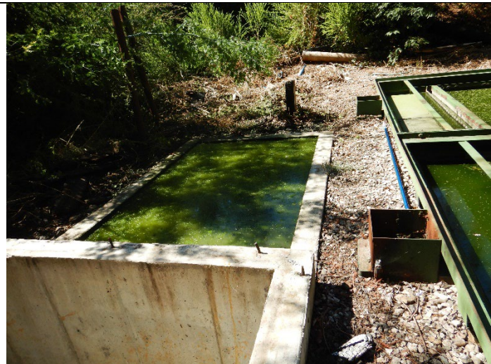
Figure 4. Basin designed for treated effluent holding untreated wastewater over basin capacity
